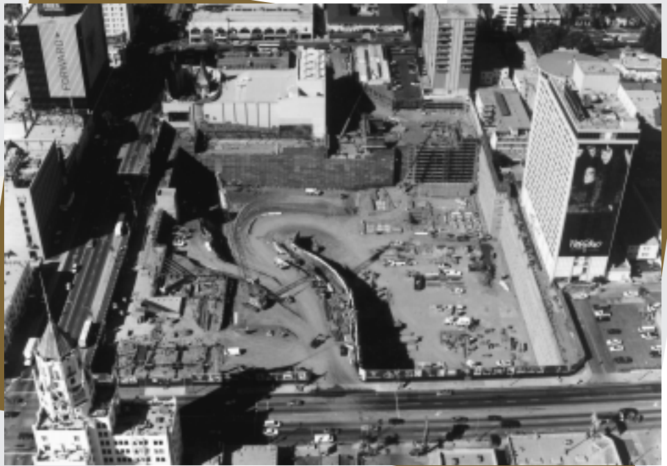
Aerial view of Hollywood & Highland entertainment center project, October 1999.
